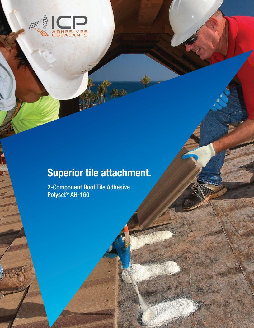
2-Component Roof Tile Adhesive Polyset® AH-160 is the professional roofer's complete solution for concrete or clay roof tile attachment. 2-Component Roof Tile Adhesive Polyset® AH-160 is a polyurethane adhesive that adheres each individual tile in place. It can be used without mechanical fasteners so it won't puncture the waterproofing membrane or roof deck. 2-Component Roof Tile Adhesive Polyset® AH-160 has superior holding power compared to nails, screws, mortar and wire tie systems.
